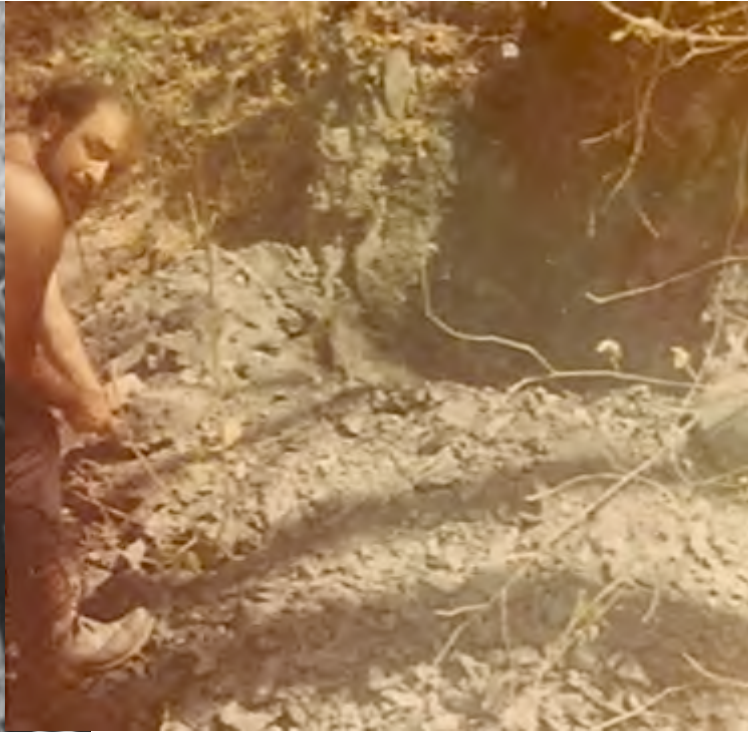
Clearing the entrance to the ventilation shaft
